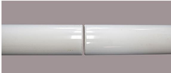
1. Chamfer and deburr both pipe ends.
