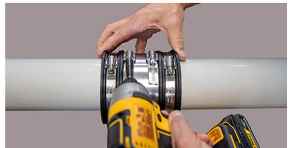
6. Center the coupling and tighten the bands.
